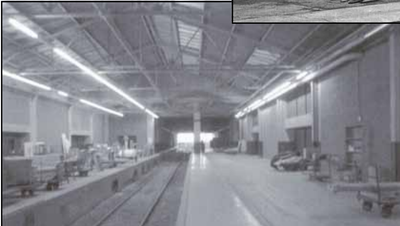
Figure 23: One of three rail spurs entering under cover at the east entrance to the building. Up to 18 freight cars could be offloaded daily on site. Loading docks lead to banks of freight elevators and a conveyor system. (Courtesy Heritage Investment Corp.)
