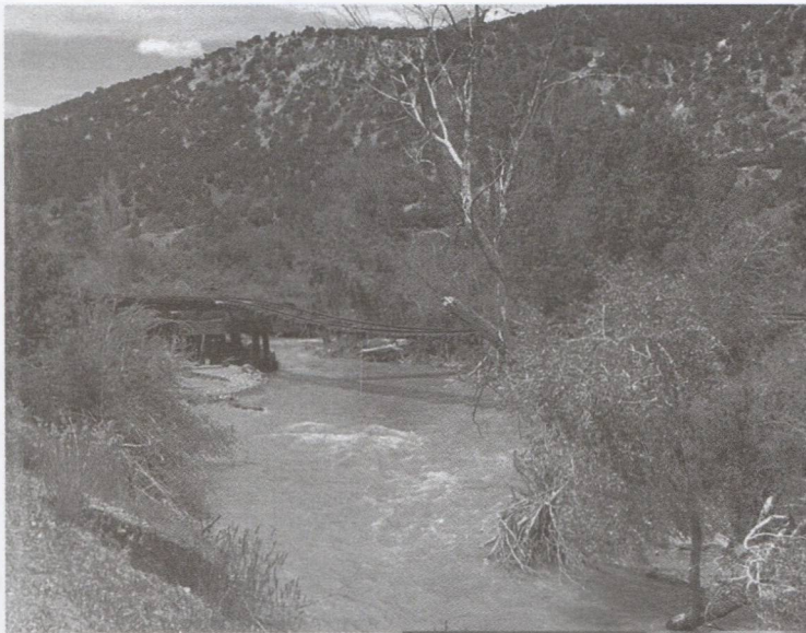
Figure 21 Bridge on Thistle Creek washed out by 1983 flood. (Courtesy of US Geological Survey.)
