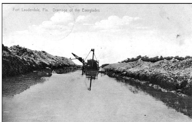
Figure 4 A 1909 view of the dredging process at Fort Lauderdale, a daily, weekly, monthly, yearly process to reclaim land.
