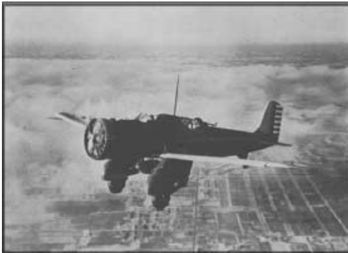
Figure 6-9 Curtiss A-12, state-of-the-art attack aircraft could carry 400 pounds of mail, and was used in the rugged northwest. Type of aircraft in which Lts. Grenier and White lost their lives in the early period of the Army emergency air mail operation.
