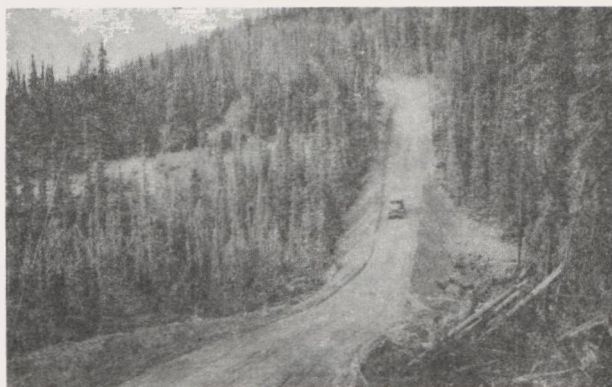
Postal view card, "Alaska Highway showing the valley filled to reduce the grade. Photo 16."
